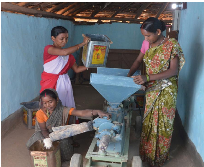
Solar mini-grid power provides electricity for grain milling Source: Mlinda, 2019
